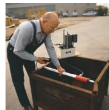
Straightening of a container box by use of a hydraulic cylinder YS-10/150, extension tube AYS-106, base adaptor AYS-103 and electric power pump PY-04/2/5/2 M.
